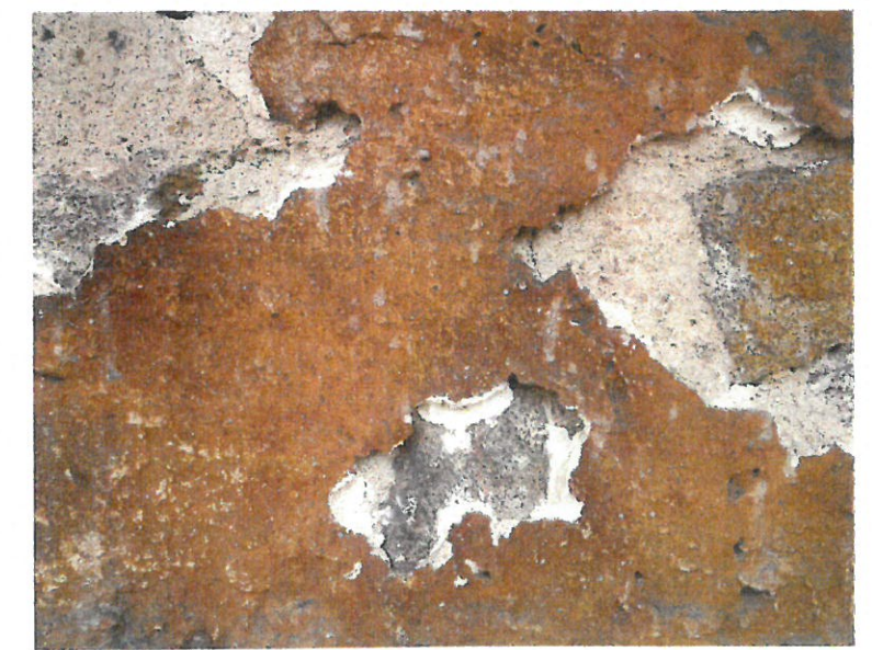
Figs. 11 and 12 (Left and below) So-called 'emergency rescue' is carried out prior to the first limewater application. It is intended to improve the render's adhesion to the substrate and reaffix delaminated material. (Photo D. Michoinová)
