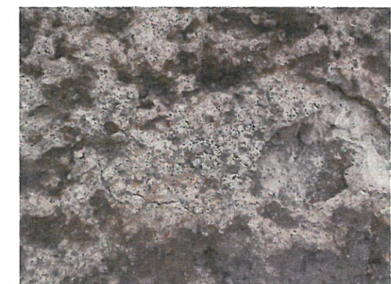
Figs. 5, 6 and 7 (Top, left and below) Historic renders that are friable and without a continuous limewash or other surface coating, which would inhibit limewater absorption, are suitable for limewater consolidation. (Photo D. Michoinová)
