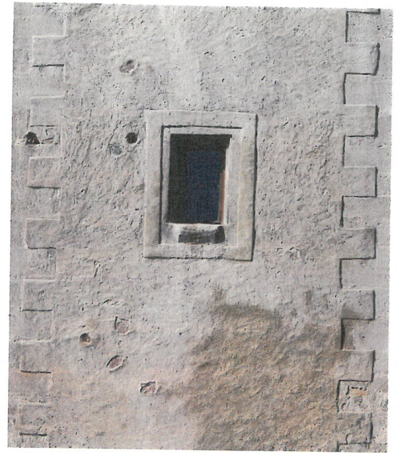
Fig. 15 (Above) Limewater is useful for pre-wetting the masonry before a new lime mortar application. It is also useful for moistening new lime materials (here a render) as part of the curing regime. The limewatering inhibits the early drying of the render and accelerates the carbonation of lime binder in the render. Here, the new lime render can be seen on the lower right, extending down part of the Švihov Chapel facade. (Photo G. Čapková, 2012)
