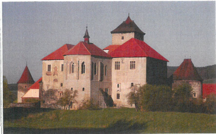
Fig. 2 (Above) Švihov Castle, Czech Republic (late 15th century). Although the castle's facades were not maintained prior to 2003, since that time their conservation has been ongoing. Limewater proved to be a very effective material for render consolidation and biocide maintenance as well as in the curing of new lime-based supplements. (Photo G. Čapková, 2016)
