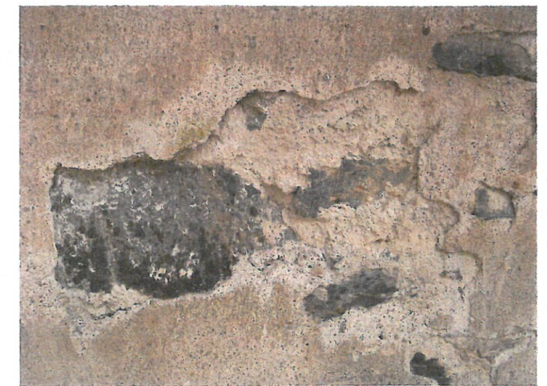
Figs. 5, 6 and 7 (Top, left and below) Historic renders that are friable and without a continuous limewash or other surface coating, which would inhibit limewater absorption, are suitable for limewater consolidation. (Photo D. Michoinová)
