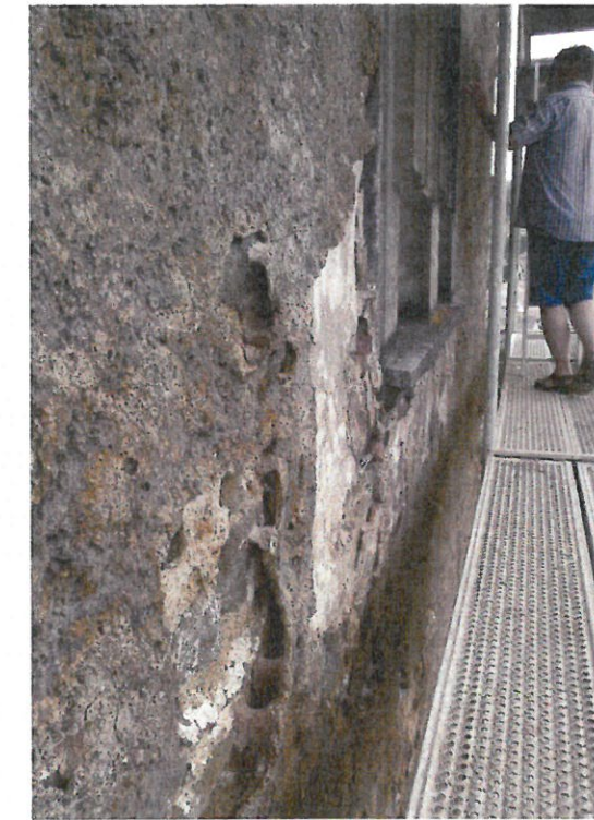
Figs. 11 and 12 (Left and below) So-called 'emergency rescue' is carried out prior to the first limewater application. It is intended to improve the render's adhesion to the substrate and reaffix delaminated material. (Photo D. Michoinová)
