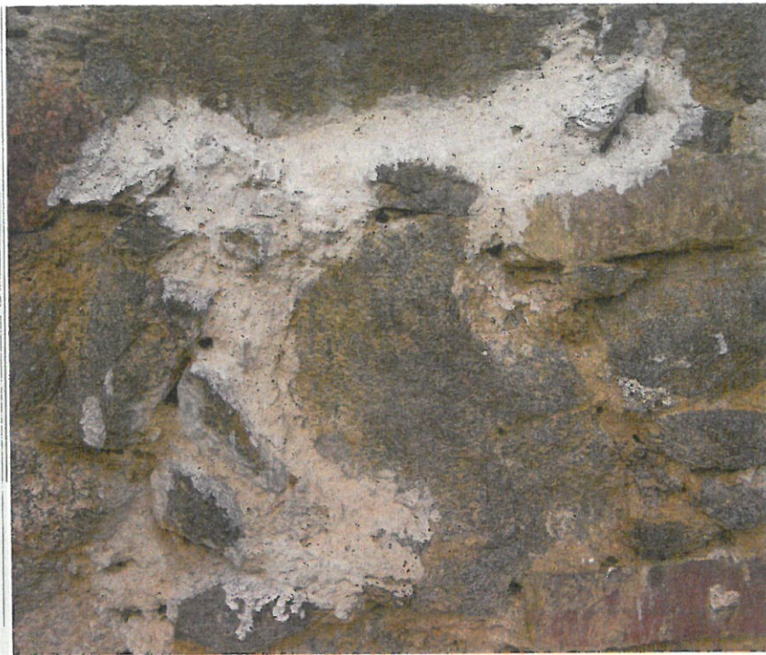
Fig. 16 (Above) This plate shows an area of friable render after the application of a suspension of lime in limewater. This is used when limewater alone is not able to consolidate the mortar, even after tens of cycles. (Photo D. Michoinová, 2011)
