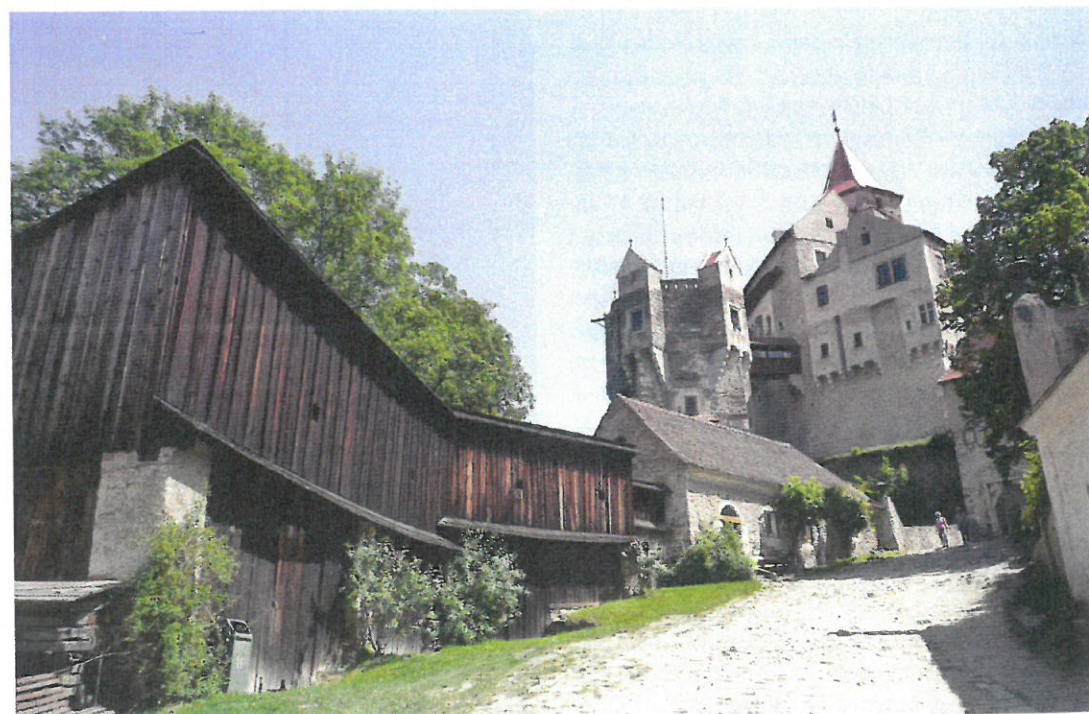
Fig. 3 (Right) Pernštejn Castle, Czech Republic (mid 13th century). In 2006 lime-rich renders on the palace were consolidated by limewater, followed by consolidation of minor areas using a lime suspension in limewater. The image shows the tower (centre) before its conservation. (Photo D. Michoinová, 2009)
